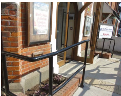
A newly added ramp and level access
