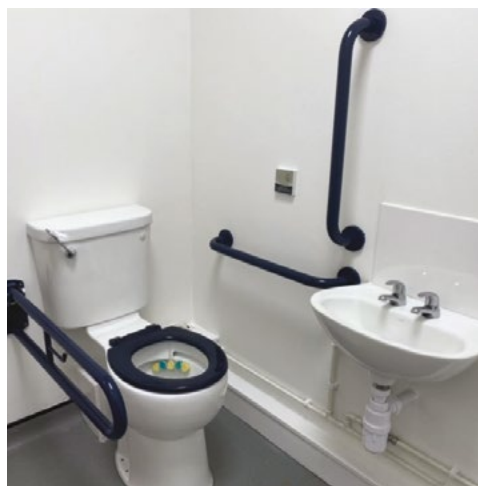
A newly installed accessible WC
