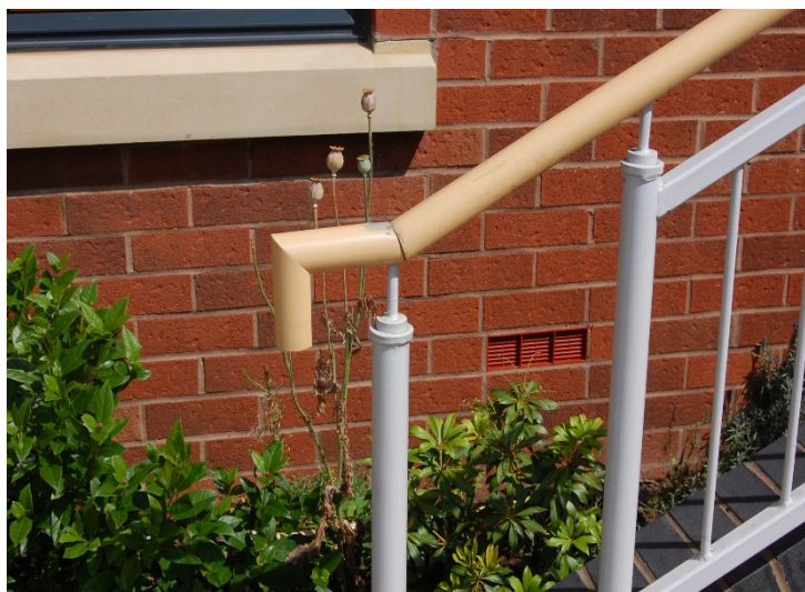
Figure 5: Vertical termination of handrail.
