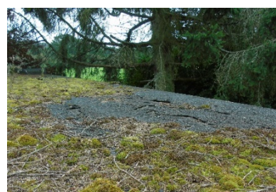
Moss and tree debris gathering on flat roof and cracking of roof
