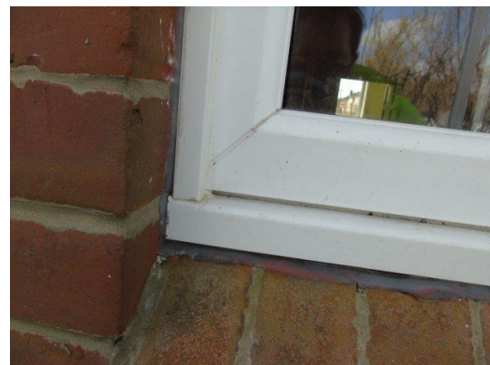
Mastic sealing around windows
