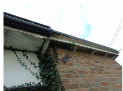
Ivy ingress and damage to external wall and soffit
