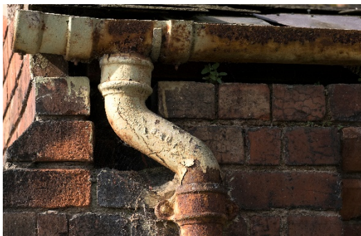
Cast iron gutter
