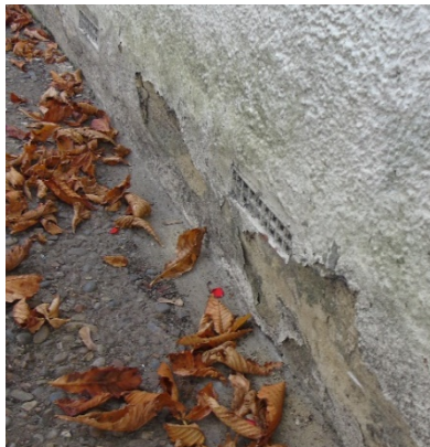
Cracking render
