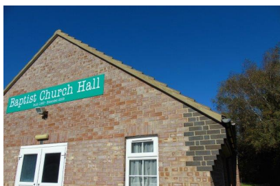
Mortar pointed verge
