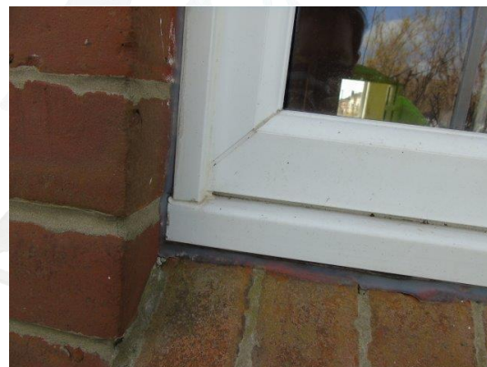
Mastic sealing around windows
