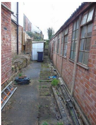
Asbestos pipe waste
