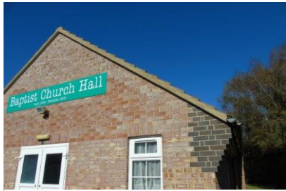
Mortar pointed verge
