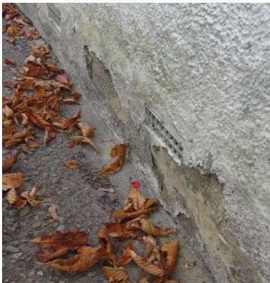
Cracking render
