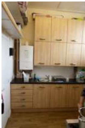
Photo 5 – new units to kitchen
