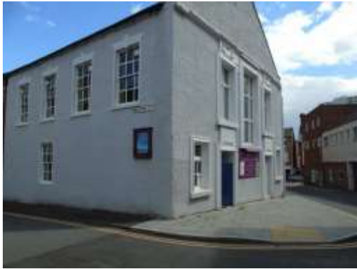
Photo 1 – front view of the Main Hall
