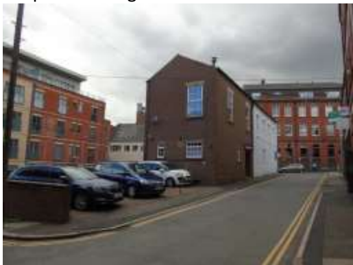
Photo 3 – building viewed from rear with car park in foreground
