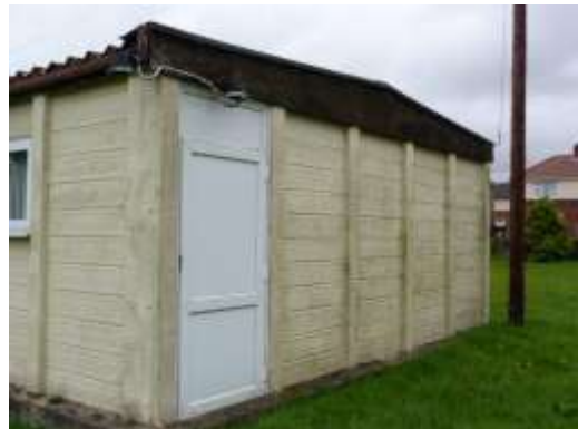
Photo 6 – rear view of main building
