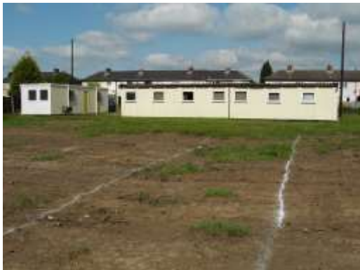
Photo 5 – side view of buildings
