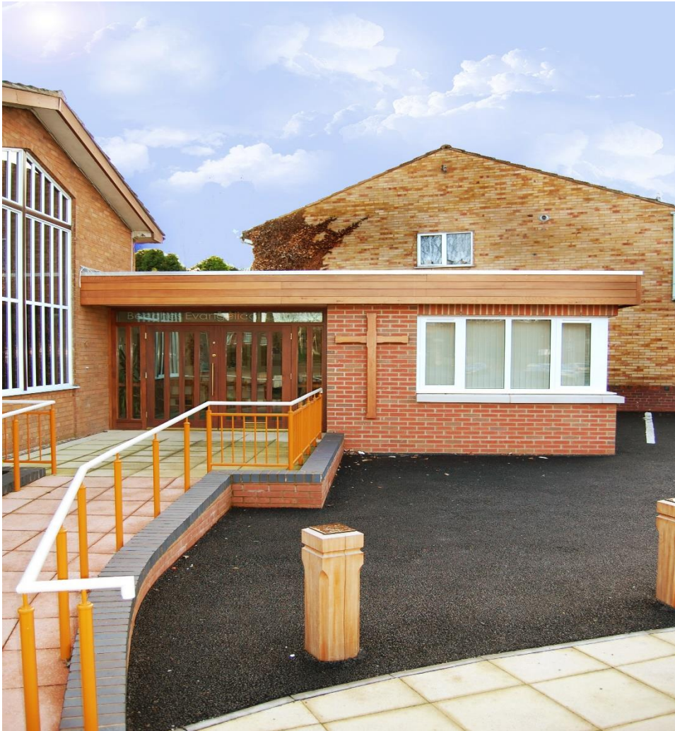
Figure 1: An example of a replacement ramp to an evangelical church in Birmingham.
