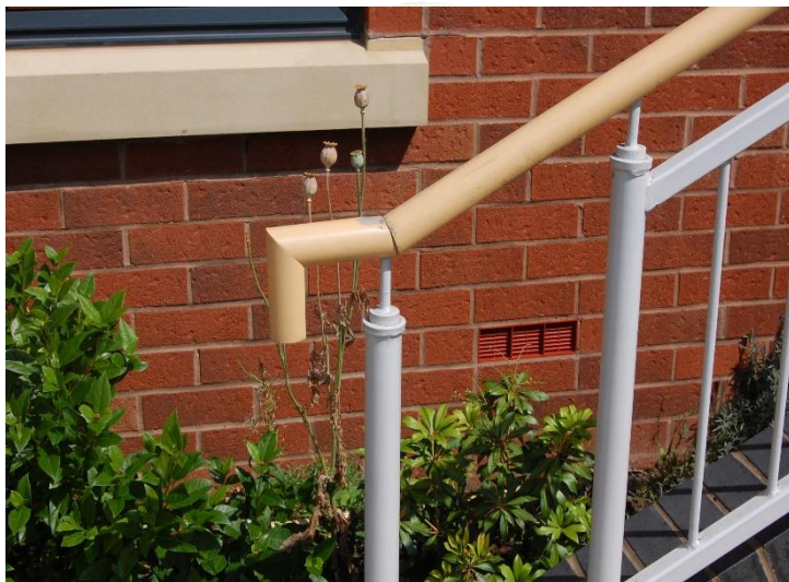
Figure 5: Vertical termination of handrail.
