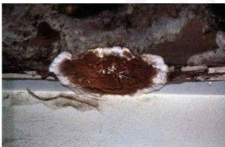
Figure 6 Fruiting bodies are fleshy and soft shaped like pancakes or brackets. When they are ready to fruit, they bear masses of tiny rusty red spores which settle on surfaces with the appearance of rust-coloured dust.
