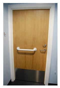
Left - Interior of the door illustrating the horizontal grab rail in line with the door handle. Also, note the deep kick plate to protect the door from damage by wheelchairs.
