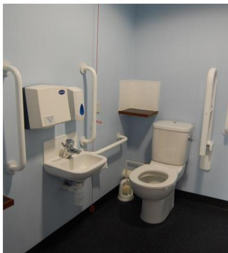
Above - examples of good tonal contrast between fittings and wall, fittings and floor & walls and ceiling.
